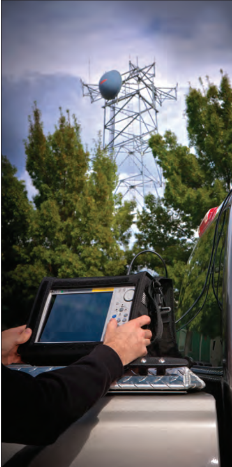
LMR Master Testing from a Service Vehicle
